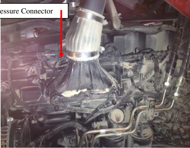
Engine Compartment in a 6.7L Puma
